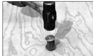
Wood Form Insert Installation Sequence
